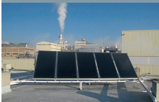
Pilot projects: In Spain, we have installed small-scale solar thermal systems at our sites in Seville and in Montornès (photo). These systems use the heat from solar radiation to provide hot water for the sites.
